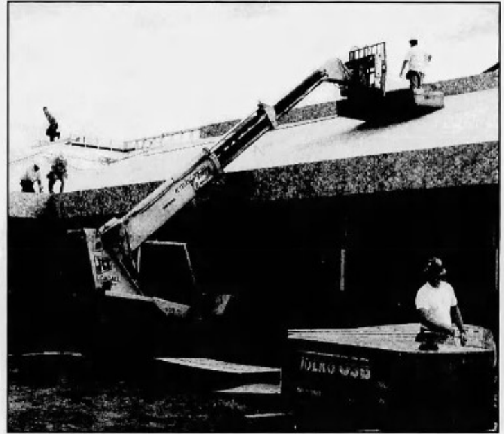
Brendan Dow (foreground) gets some roofing material ready to hoist over rafters at the Lions Learning Centre. With construction well under way project organizers are looking forward to the building's completion by November.
